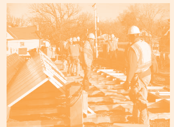
Jon Kramer and his associates at Sundial Solar installed a 20 kilowatt passive solar array on the co-op's roof in October of 2010. The panels were manufactured in Minnesota by TenK Solar. The panels are estimated to provide 5-7% of Eastside's annual electricity needs.
